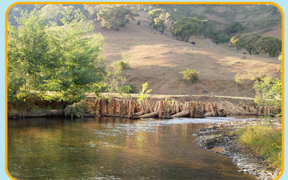
Recent habitat works on Nariel Creek
